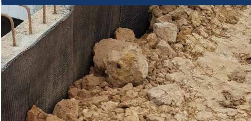
TerraDrain® is a dimpled plastic sheet that provides effective drainage and waterproof membrane protection on foundation walls and other underground structures. The integrated non-woven geotextile covering the dimples prevents soil particles blocking the drainage sheet, creates an air gap for reliable ventilation and allows inflow and with its dimple structure effectively captures and transports high water volumes and resists high loads from earth and formwork.
