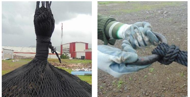
Once knotted through the steel ring, the FRN Gabion is safe to be lifted using the same ring. The filled FRN Gabions can be directly installed using lifting equipment or transported and installed in required sites. Ensure safe working conditions at all times.
