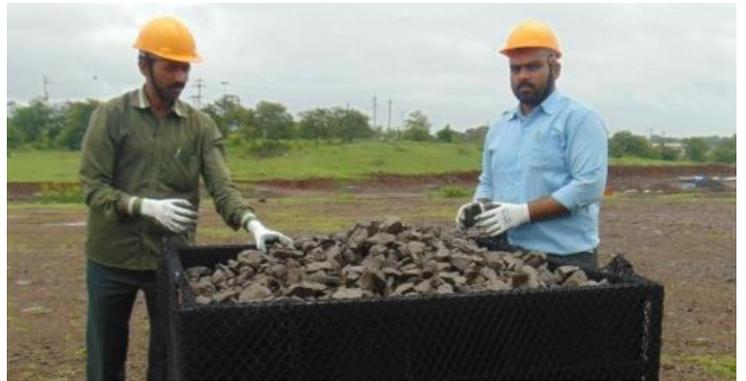
After filling is completed, close the ropes and bind the net with rope as shown here. Pass all the overhand ropes through the steel ring provided and knot it
